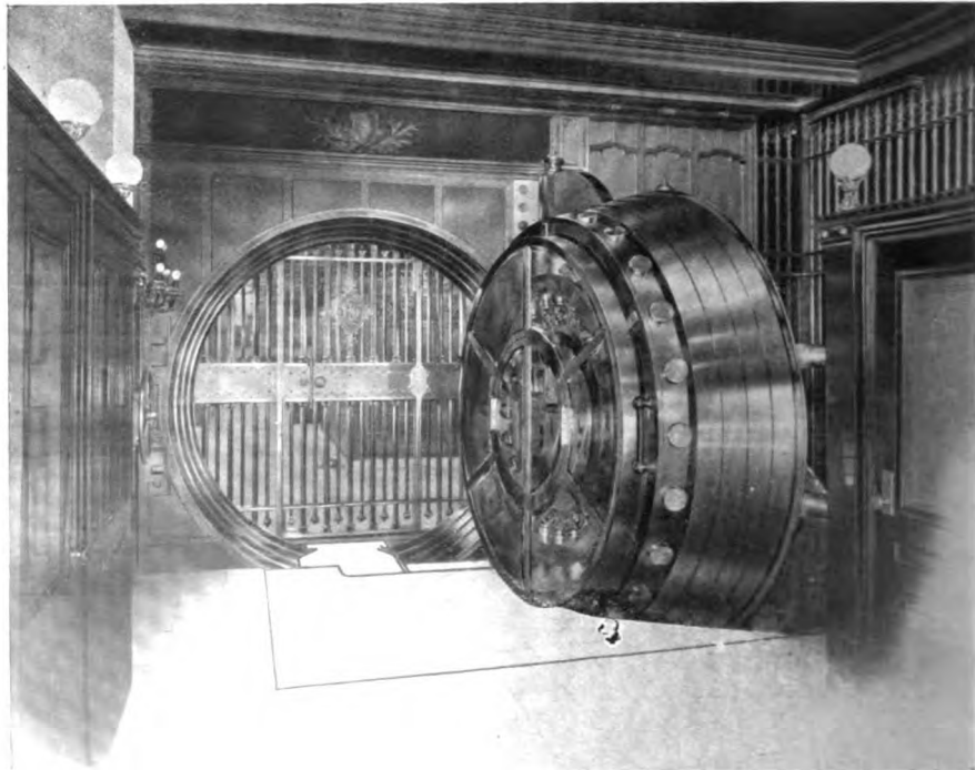
ONE OF THE 25-TON DOORS
